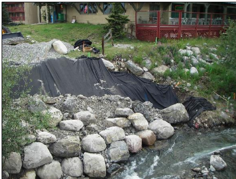
Figure 4.3. Filter fabric installation example
